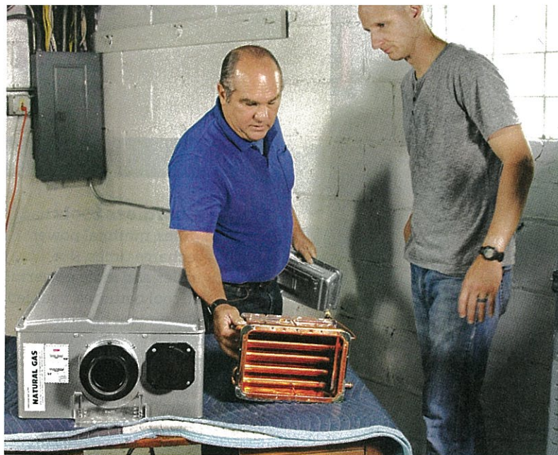
LEFT: Richard Trethewey explains how the copper heat exchanger in a tankless water heater transfers the heat from a gas flame to the water flowing through the tubing.
